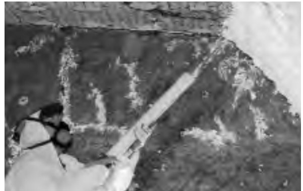
Projection d'Isofoam/Foamfrax
